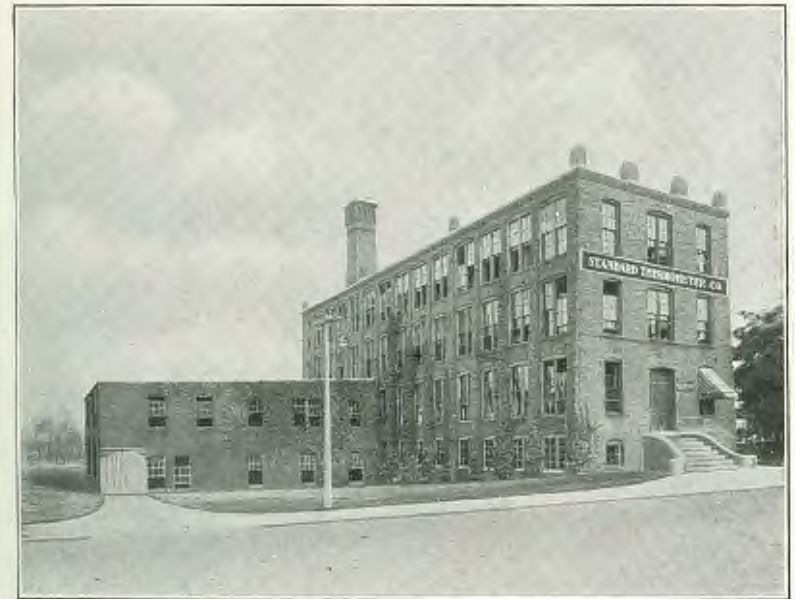
Main Office and Factory No. 1.
